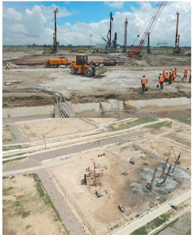
Soil Mass Stabilization Work at Industrial Base Under Unit 1
